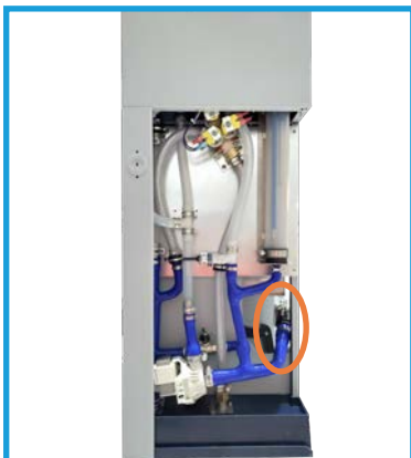
Disconnect the water inlet
